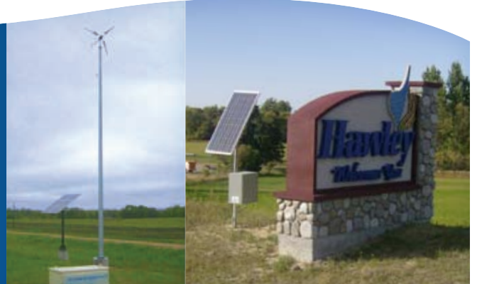
Off-grid renewables may be less expensive than bringing in utility lines.
